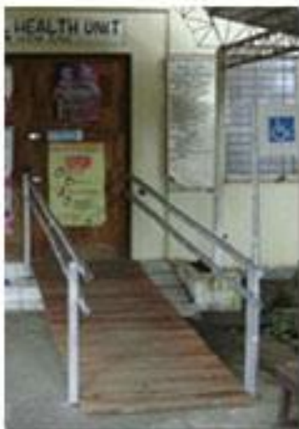
Barrier-free and accessible structures for persons with disabilities such as ramps, hand/grab rails, and signages, among others, have become familiar sites in the NHE pilot areas.
