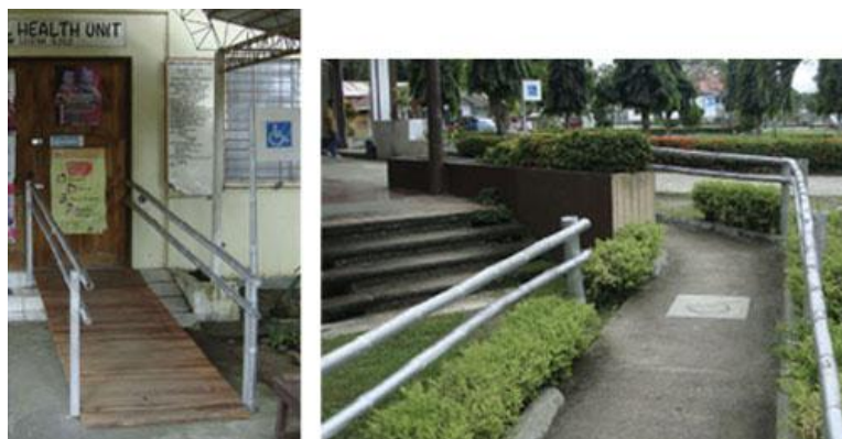
Barrier-free and accessible structures for persons with disabilities such as ramps, hand/grab rails, and signages, among others, have become familiar sites in the NHE pilot areas.
